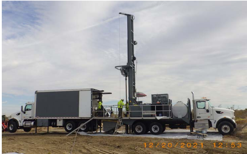
Terrasonic 600 drill rig
