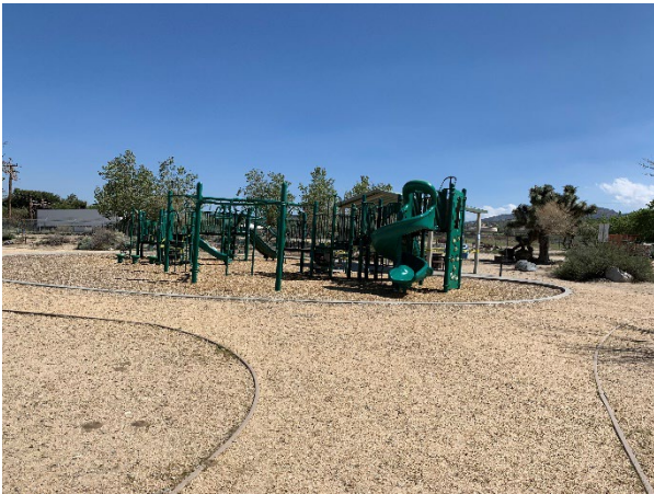
Existing Playground Structure
