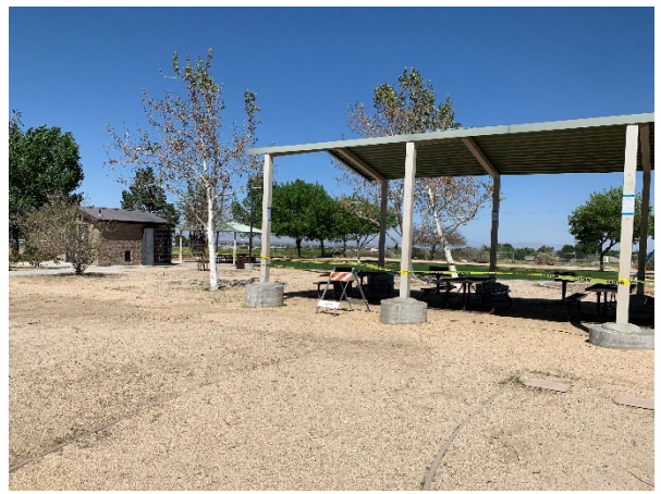
Existing Picnic Structure
