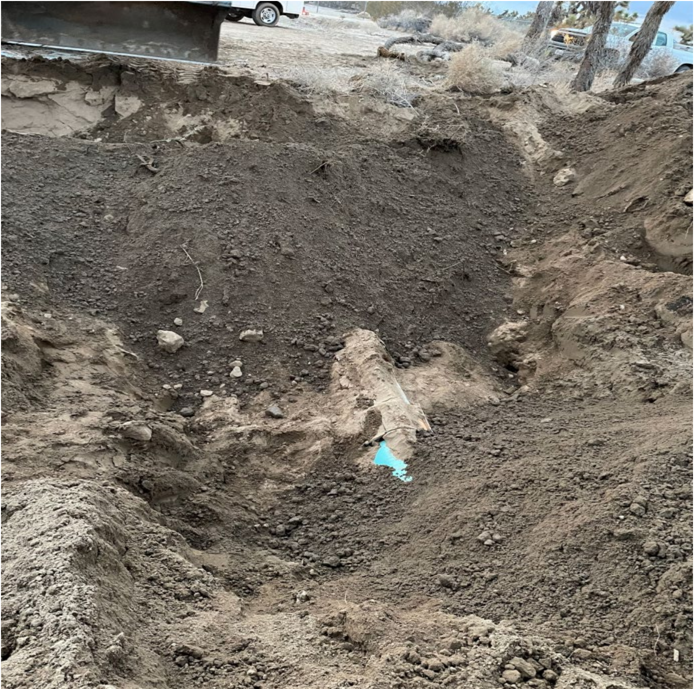
Well 14 16" Mainline repair
